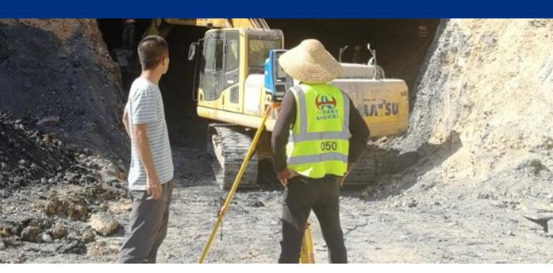
**Huizhou City, China (April 2018)**— FOCUS 35 robotic total stations are hard at work helping build the world's largest expressway network. In one notable example, the FOCUS 35, with its time-saving automatic scan template, is checking the cross-section quality of the twin Nan Kunshan tunnels for the new six-lane Shazhan S14 regional highway.
