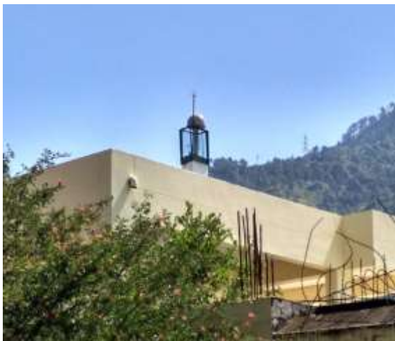
CORS STATION HNBGU SRINAGAR
